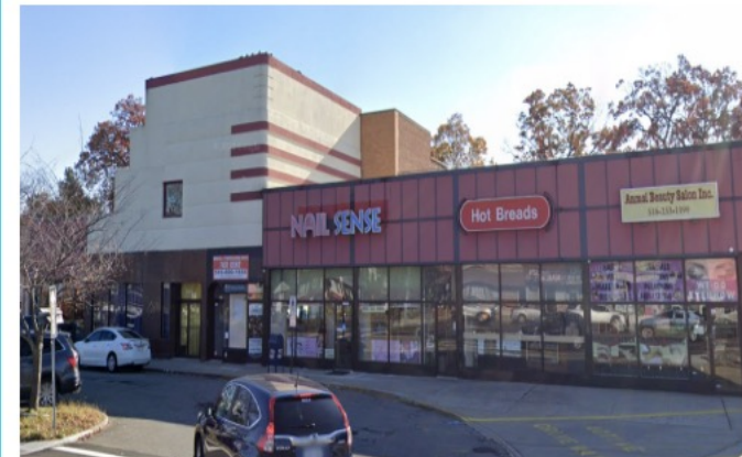
1614 Hillside Ave New Hyde Park, NY
